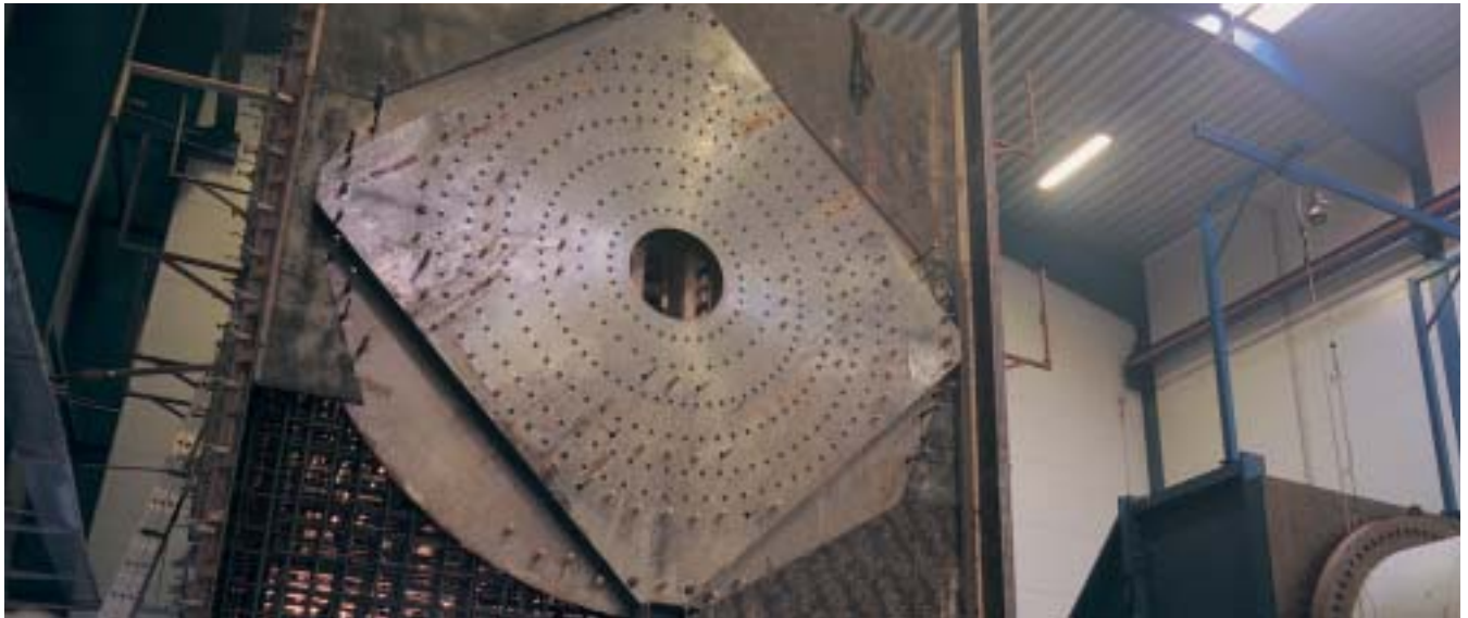
Building a structure that meets the requirements for testing very large blades is quite a challenge
