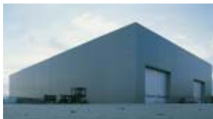
LM Glasfiber has extended its test hangar and increased the capacity for testing large blades
