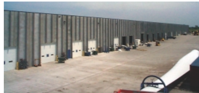
The new extension adds 3500 m 2 to LM Glasfiber's existing facilities in the US.
