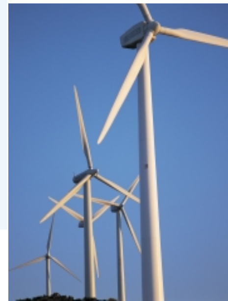
There are currently 24 turbines on the wind farm, of which 20 are fitted with LM Glasfiber blades
